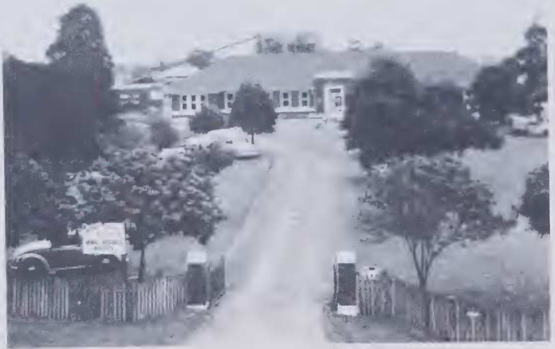
FIG. 12. Veterinary School building at Yeerongpilly, now A Block of the Animal Research Institute, Queensland Department of Primary Industry. (Animal Research Institute historical material).
